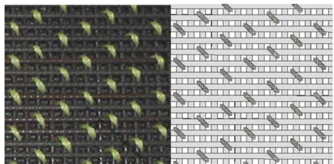
Figure 7. (a) Rebar and lacing arrangement (b) FE model
